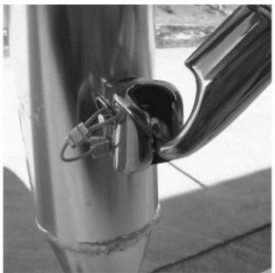
Two screws in each base attach it to the tower. The lower screw is 2" above the weld line at the bottom of each tower leg.
